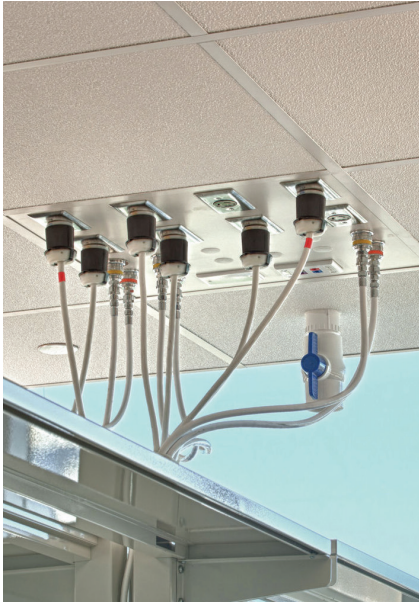
Ceiling Interface Panels [CIPs] are configured to the exact requirements of your lab; with the ability to accommodate future expansions.
